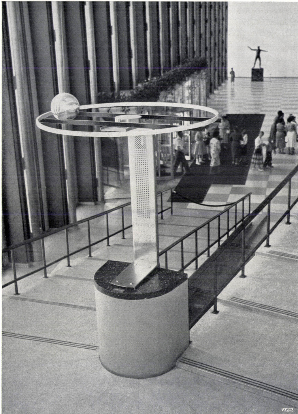
Fig. 5. The pedestal, designed by architect G. Rietveld, on which the drive coil is mounted. The pedestal bears the inscription:
